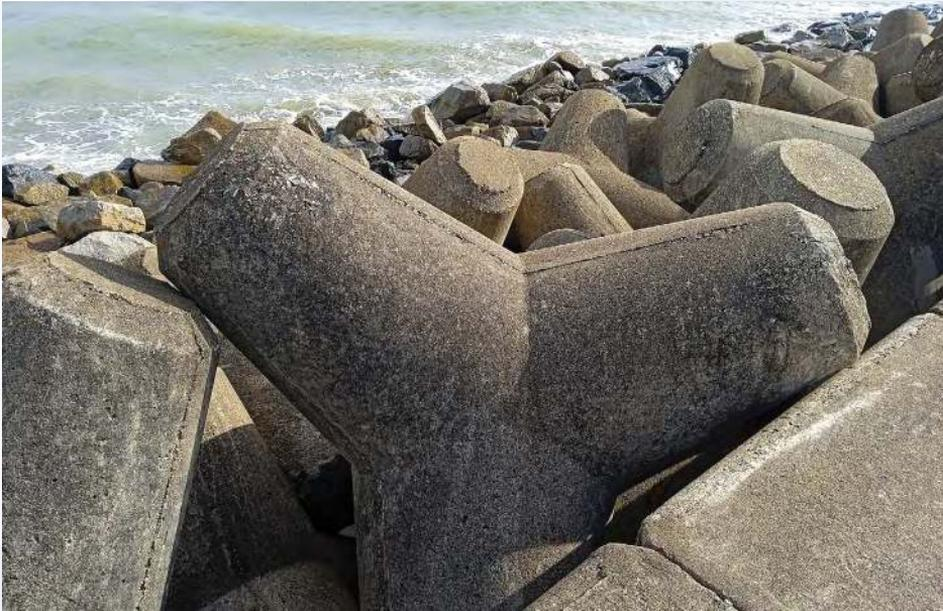
**Gambar 4.52** Breakwater
